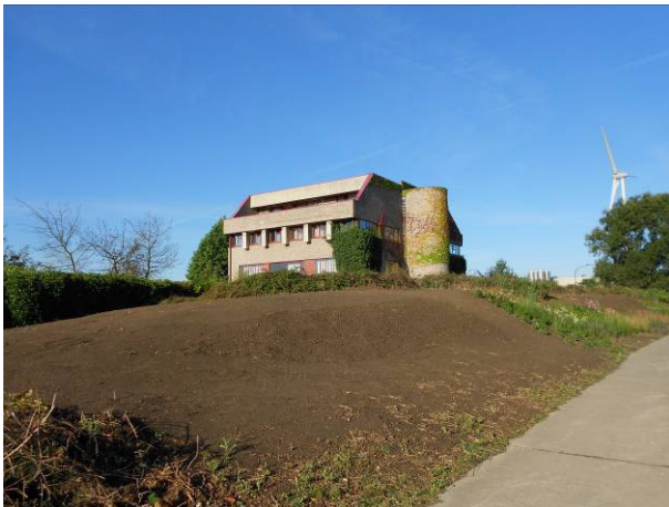
1. Date: 28/08/2012 Preparation of the slope
